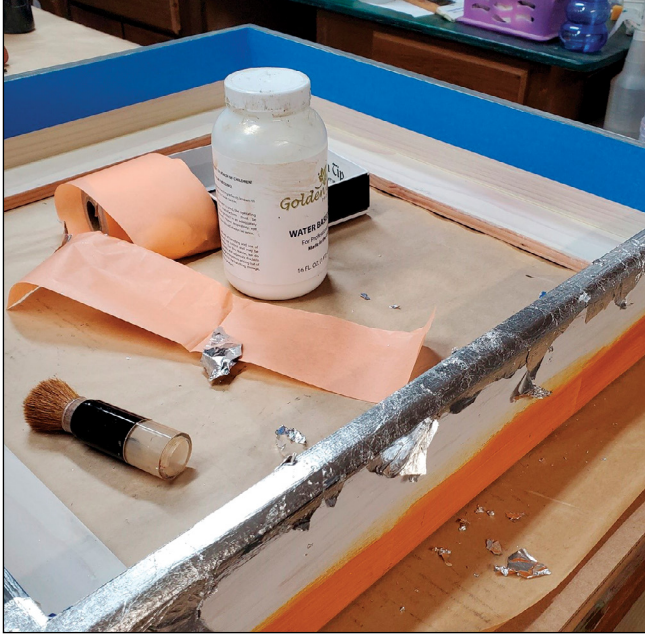
● Detail of silver leaf applied to the shadowbox to match the sample moulding.
