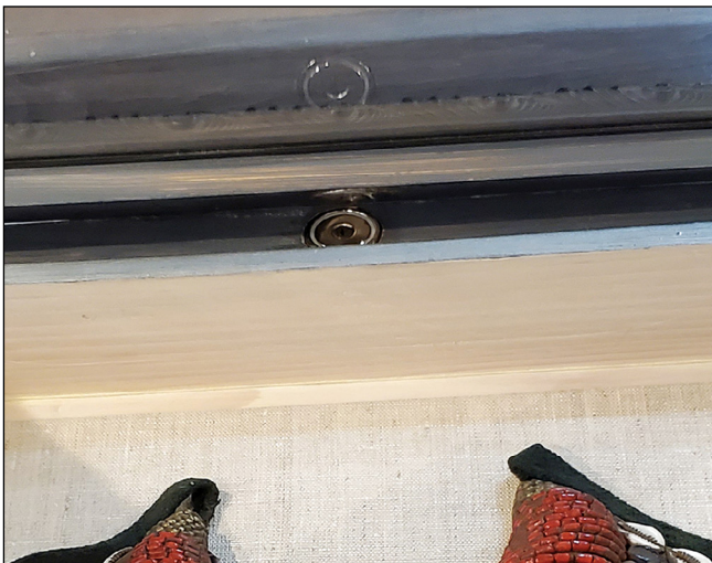
● A single recessed magnet at the top edge of the base moulding and top moulding.
